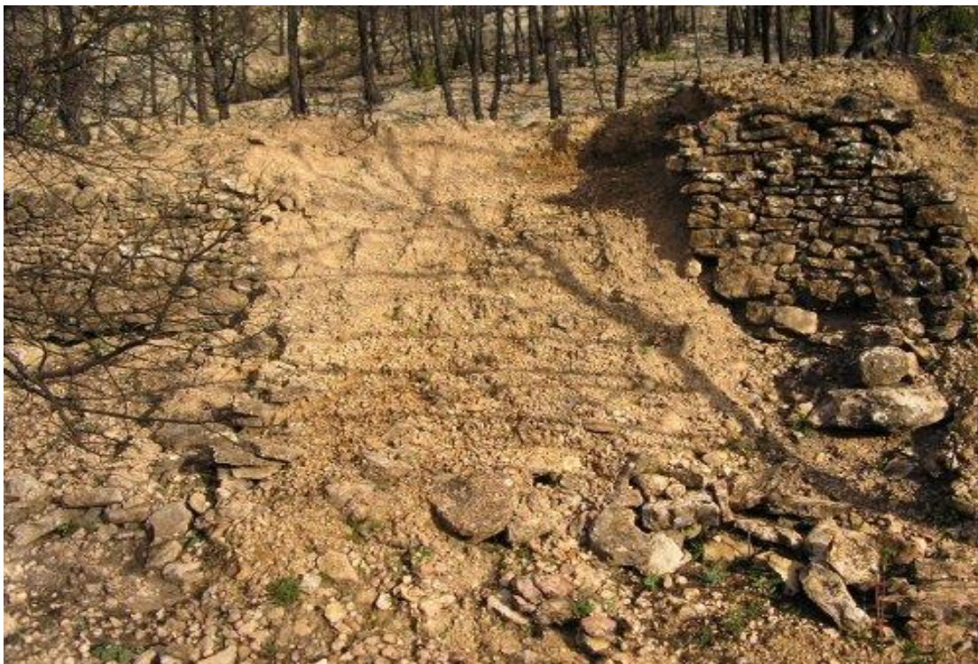
Figure 6.- Collapse in the stone-wall of a terraced plot in Bellaguarda (Lleida). Previously used for agriculture, the plot was abandoned in the 1960s-70s, natural regeneration of Pinus halepensis developed, but a wild fire swept across the area in the summer of 2005.
